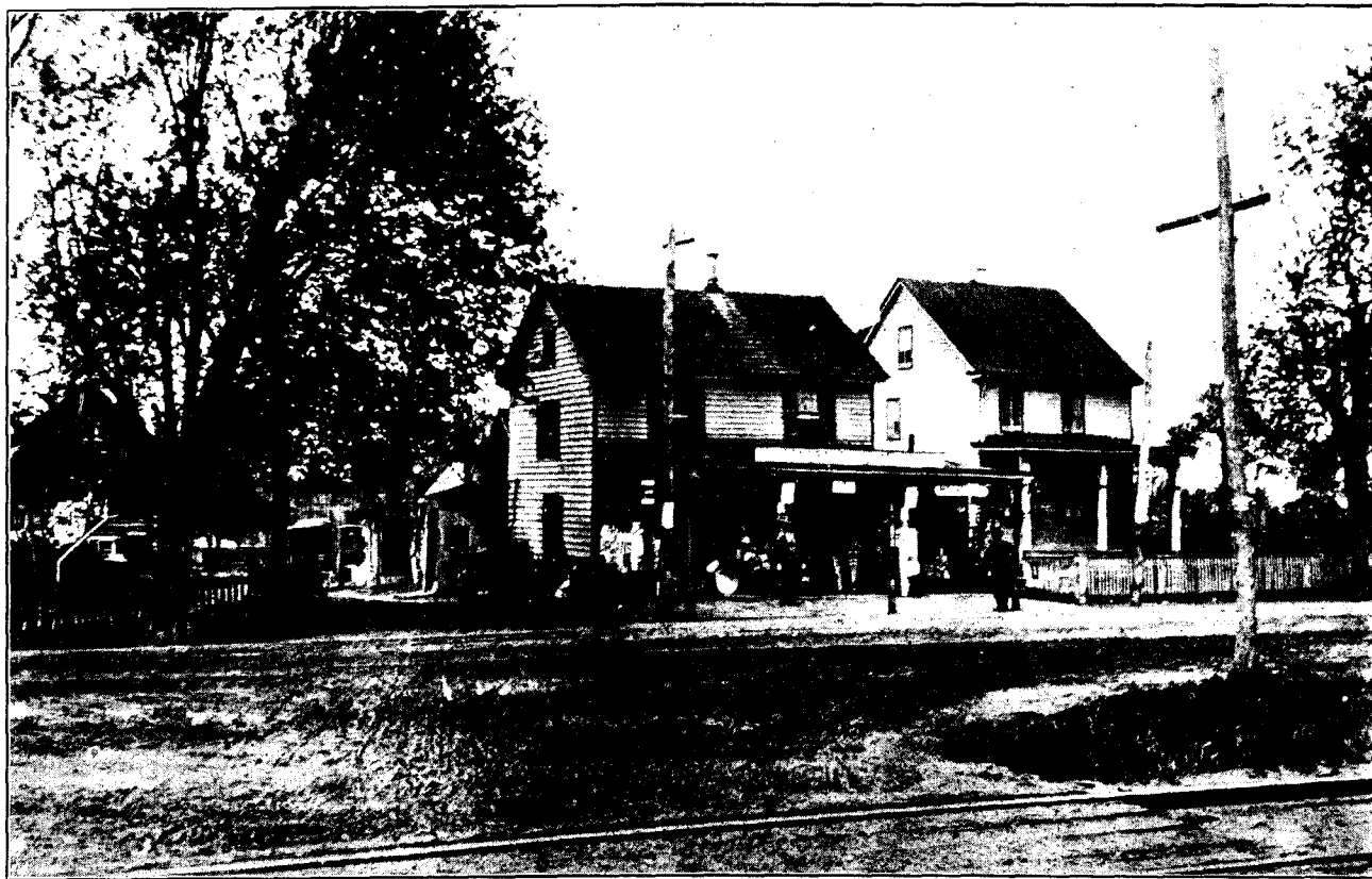
Cedar House at Masonville, N. J. Built 1682.
